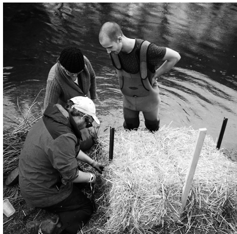
Positioning straw bales in place
